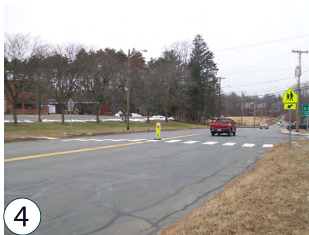
4 Wide road creates very long crosswalks in front of school.
