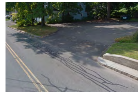
The west side of State St. is a linear gap in pedestrian connectivity downtown
