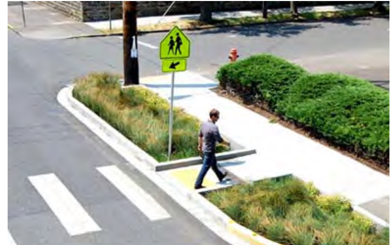
Future curb extensions on Main Street will need to be carefully designed to ensure good drainage and can potentially include stormwater retention features.
