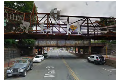
Existing conditions, looking west
