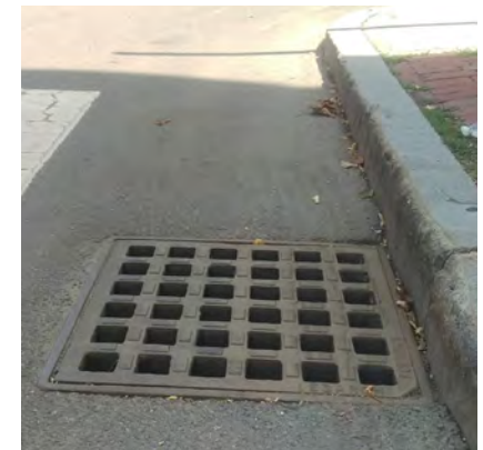
A bicycle-friendly sewer grate in Cambridge, MA. Note the direction of travel and the small opening size.
