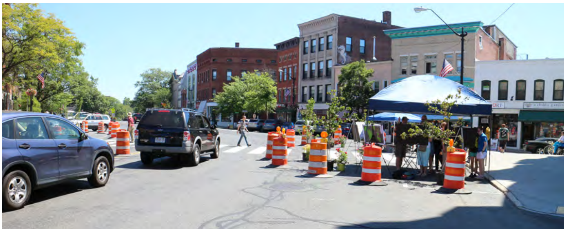
Views of the demonstration project set up that expanded the sidewalk space in front of City Hall and reduced the length of the crosswalk.
