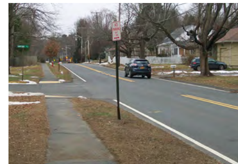
Most sidewalks outside of downtown are five feet wide with grass strips between them and the adjacent roadway
