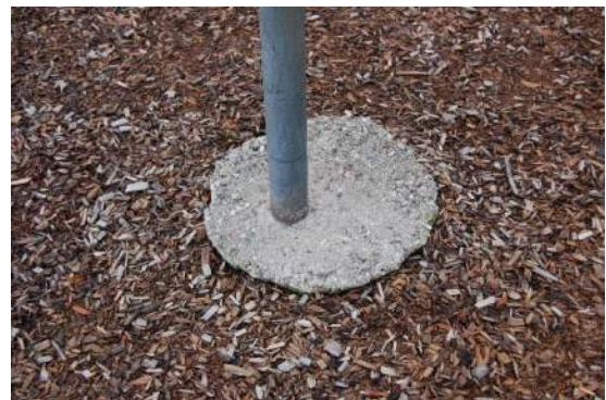
Photo 4: Exposed Post Foundation
