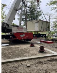
Installation of new 36" Pressure Reducing Valve building
