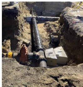
New water main installation on Damon Rd. at North King St.
