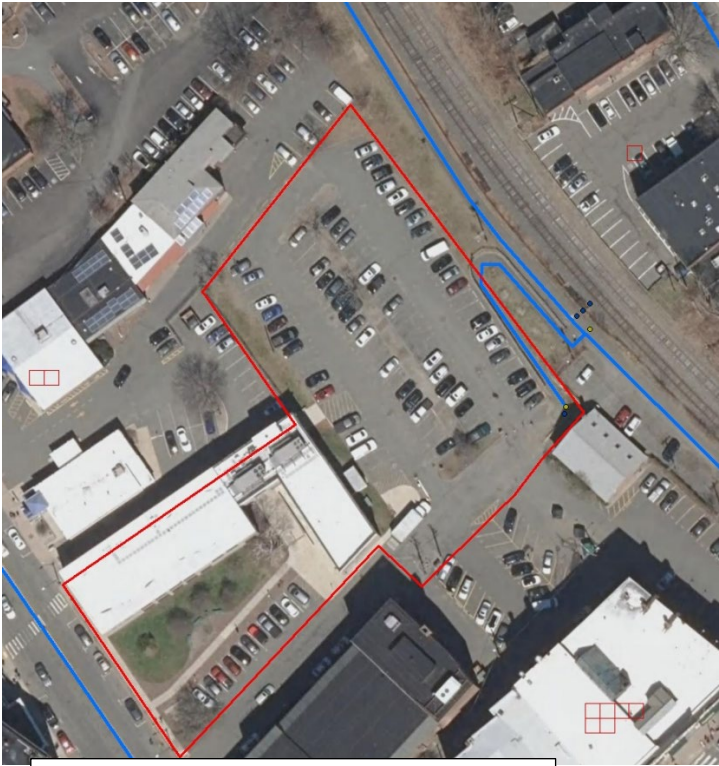
Aerial Photo of site outlined in red
